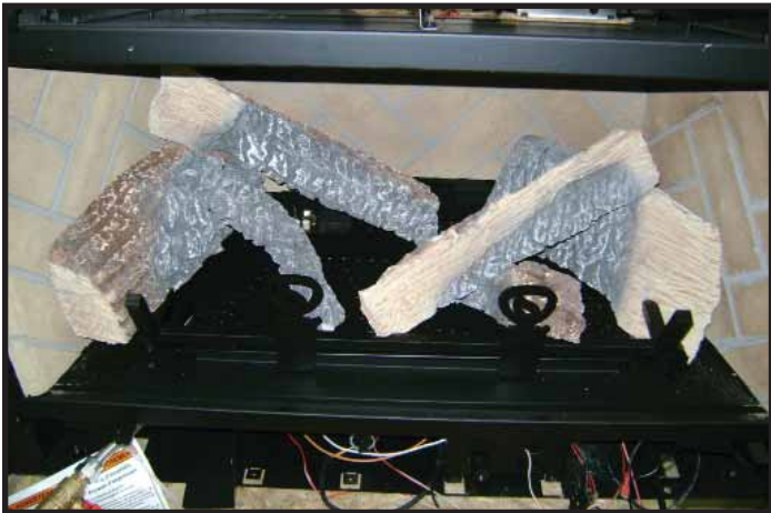
Figure 2. Refractory and Logs Installed
